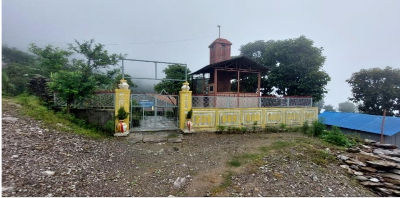
Incinerator building & main gate.
